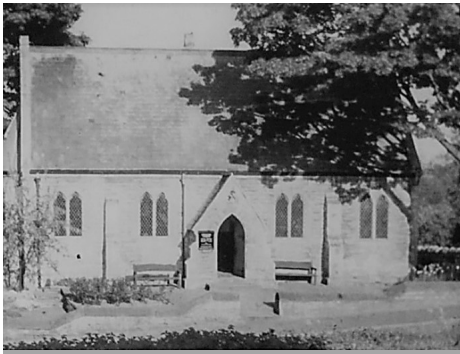
Linton School and Church
